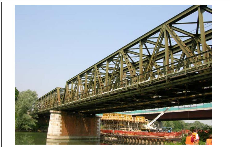
Figure 7 metal truss bridge on Brenta river
