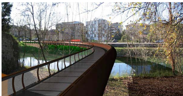
Fig. 27 View of the bridge in the context
