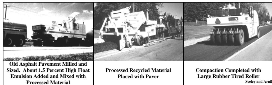
Photograph 1 Typical 1993 Ontario Highway Cold In-Place Recycling (CIR) With Emulsion Project
