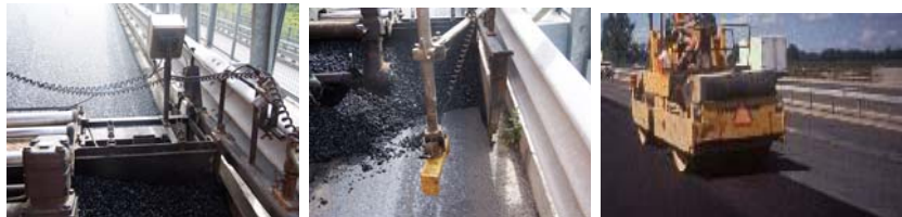
Figure 4 Hot lane compaction
