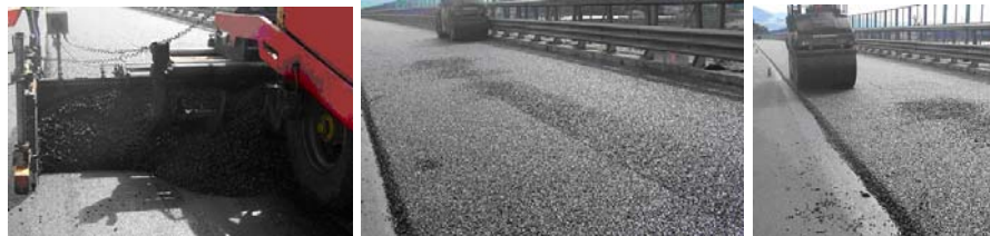
Figure 3 Cold lane compaction
