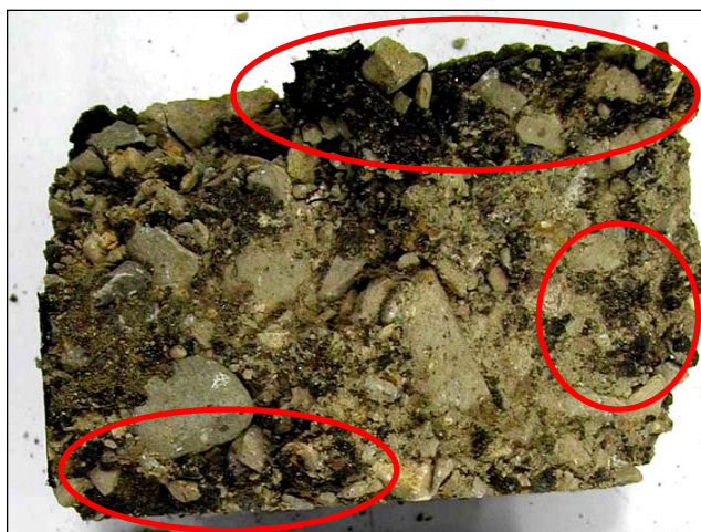
Figure 6 : Localized areas of bitumen
