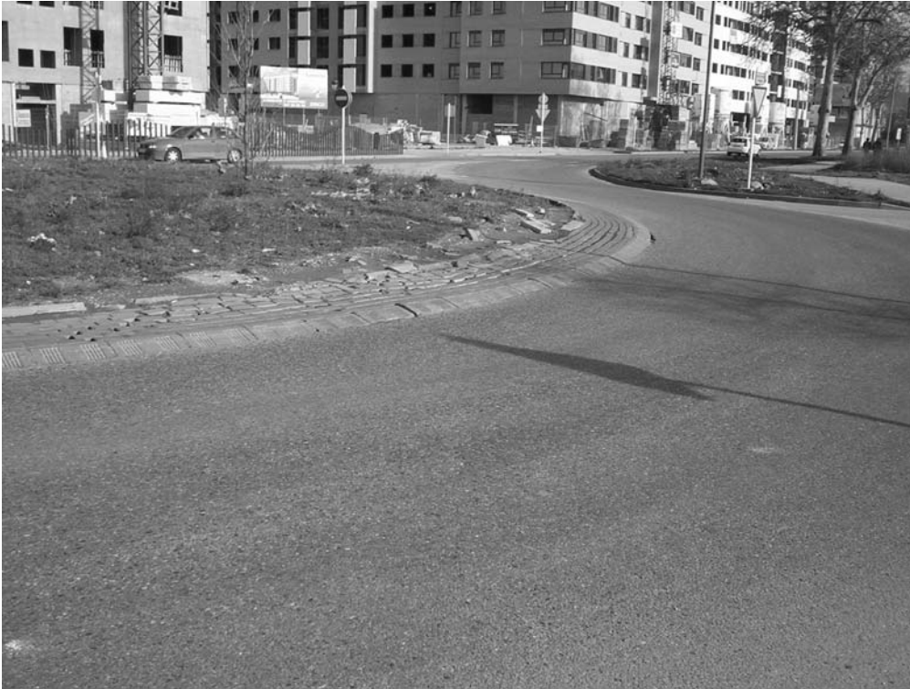
Figure 2: Roundabout with inappropriate size to support all movements of vehicles that cross it?
