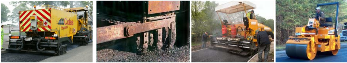
Figure 3 Repave process: heating, scarifying, laying and compaction
