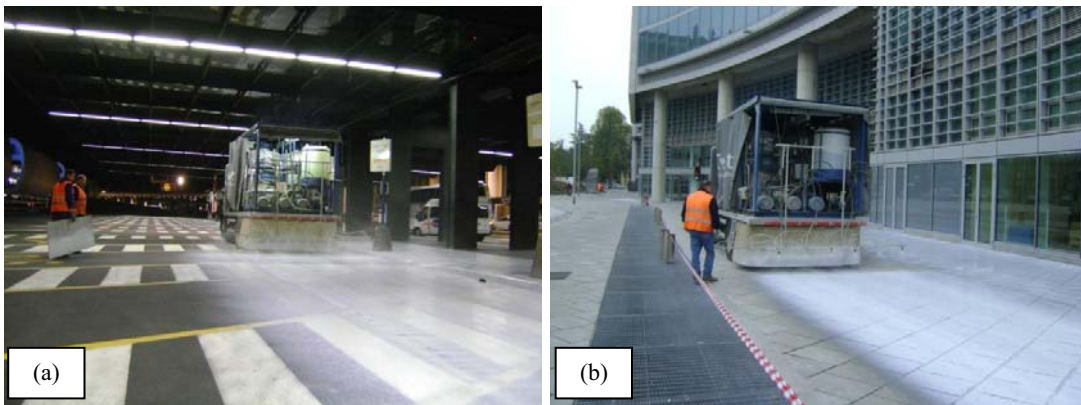
Figure 2: The application of the photocatalytic emulsion: a) Arrival area of MXP Airport (b) Viale F. Restelli in Milan's urban centre
