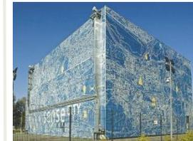
**SENSE - CITY**: "climate mini-city", is a vast reconfigurable mobile hall of 400m<sup>2</sup> capable of hosting, under controlled environmental conditions, realistic urban scenarios.
