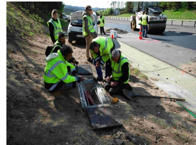
Instrumentation of pavement section on A75 in CCLEAR Project (2012)
