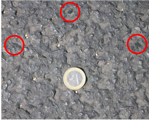
Figure 5.4: SSCR pavement surface
