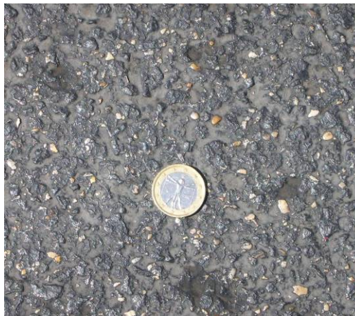
Figure 5.13: EC pavement surface
