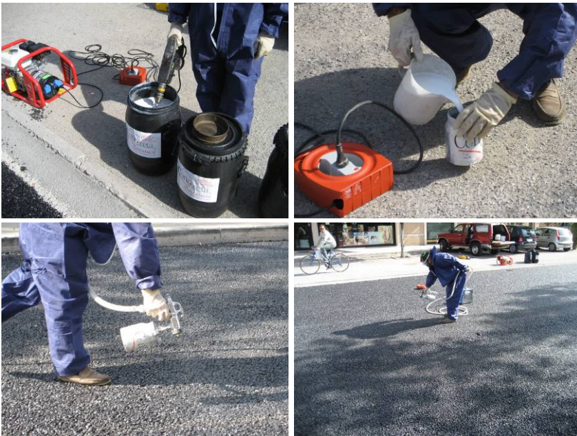
Figure 8.2: Application of the photocatalytic spray product
