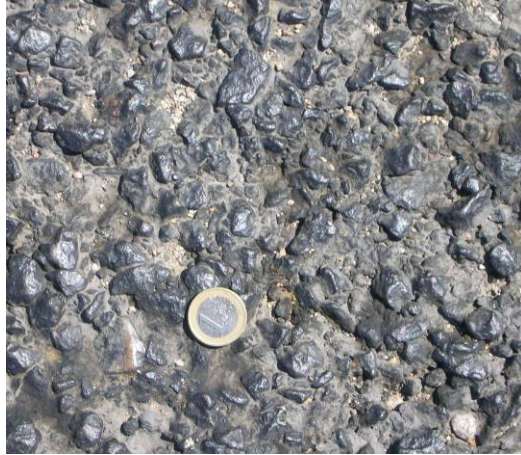
Figure 5.7: PA ravelling
