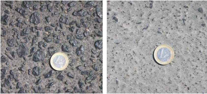
Figure 5.10: PM surface with and without mortar removal
