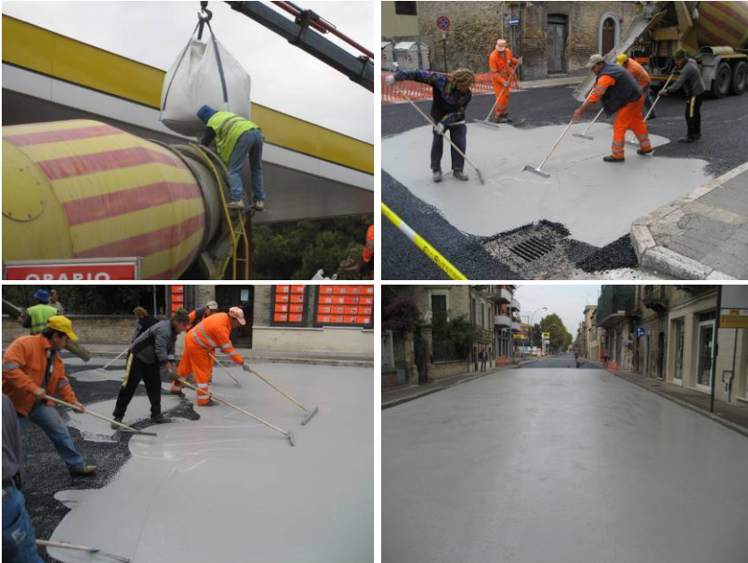
Figure 8.1: Application of the photocatalytic cement mortar
