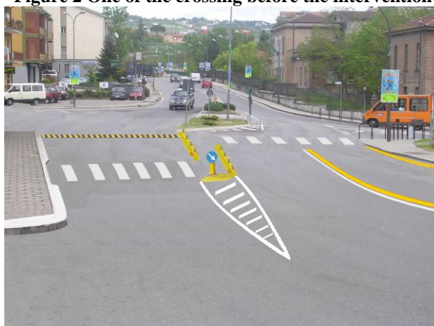
Figure 3 The same crossing after the intervention suggested
