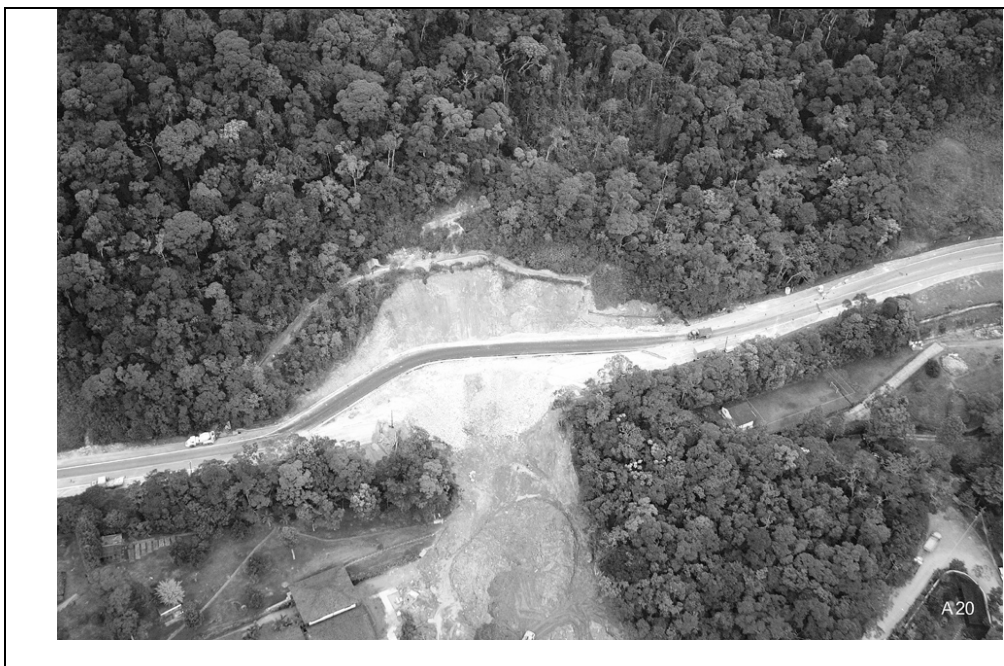
Figure 1 – A view from the land sliding location, already with a detour for temporary traffic
