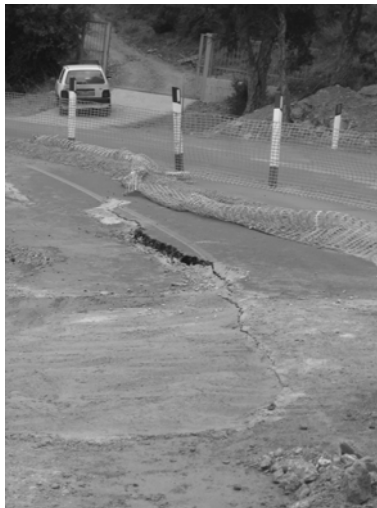
Figure 6 – Signs of the slope failure along the Provincial Road 11
