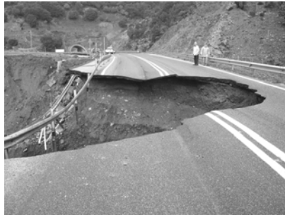
Figure 3 – Embankment collapse caused by the culvert failure.
