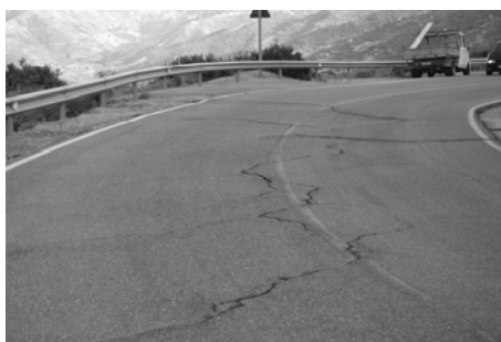
Figure 2 Initial failure of the fill slope in the State Road 198
