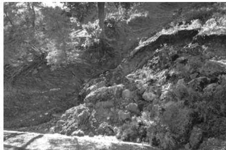
Figure 4 – Slope failure after a meteorological event
