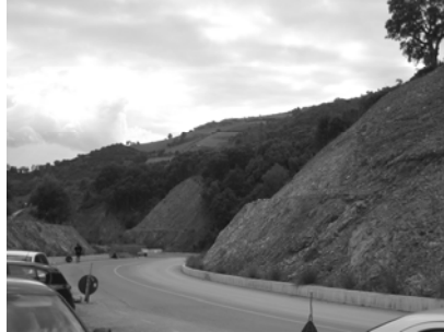
Figure 1 – Cut slopes along the S.P. n° 11.
