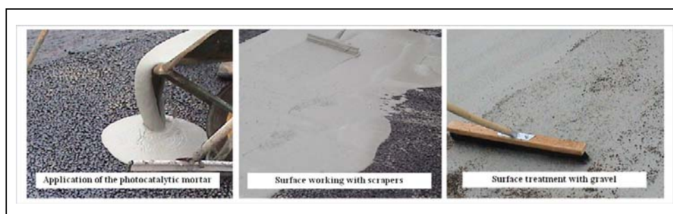
Figure 7 Application of the mortar on the pavement and surface treatments
