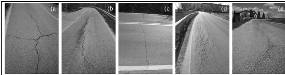
**Figure 1 Structural defects examined in this study: a) transversal and longitudinal cracks, b) longitudinal cracks only, c) transversal cracks only, d) ramified cracks, e) failures.**
