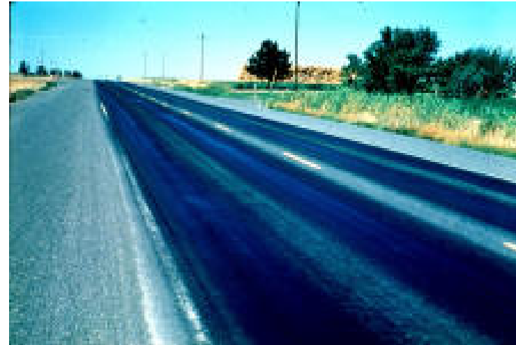
BST bleeding in wheelpaths
