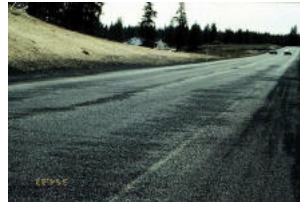
Raveling from snowplot operations
