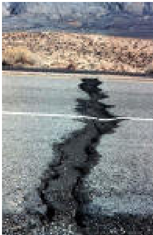
Large patched thermal crack
