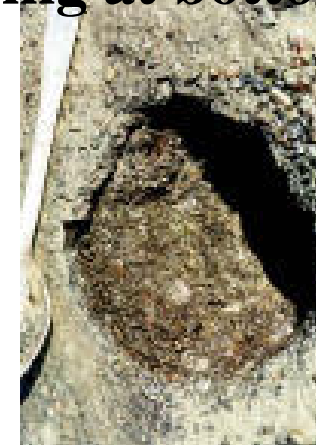
Stripping at bottom of hole
