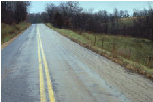
Fatigue cracking from edge failure.
