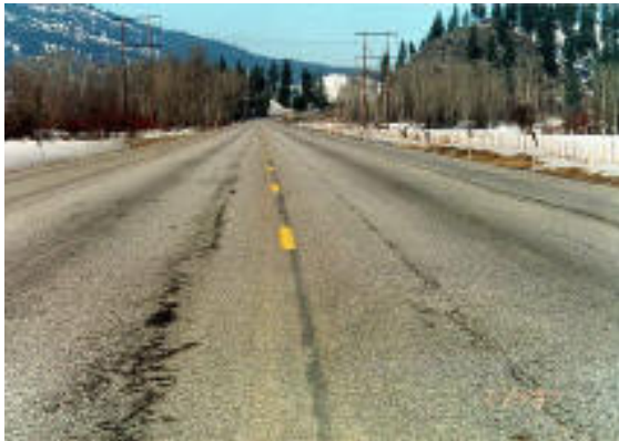
Raveling due to low density
