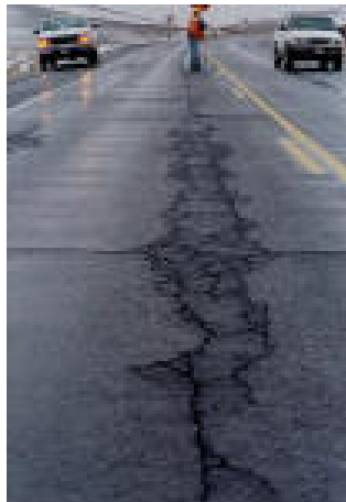
Fatigue failure from stripping; this photo shows the surface effects of underlying stripping.
