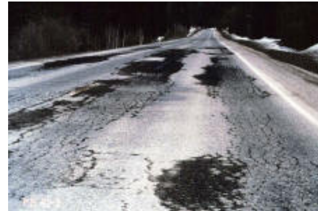
Fatigue cracking from frost action;
