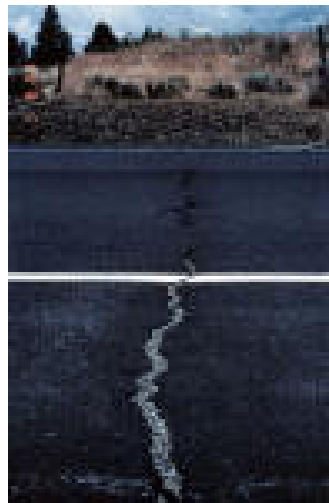
Smaller patched thermal crack
