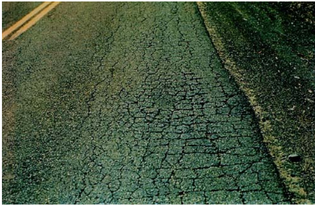
Bad fatigue cracking
