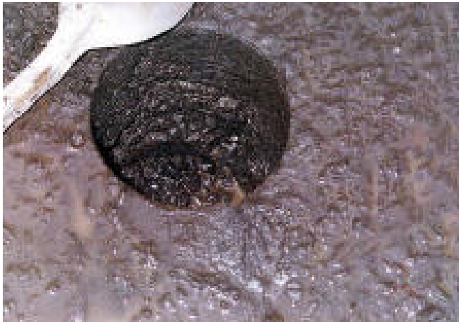
Core hole showing stripping at the bottom
