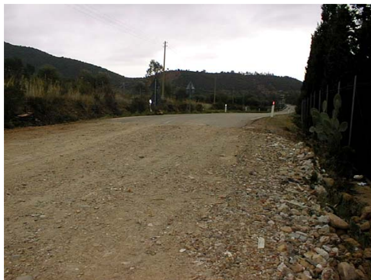
Figure 4: Foundation layer after compaction
