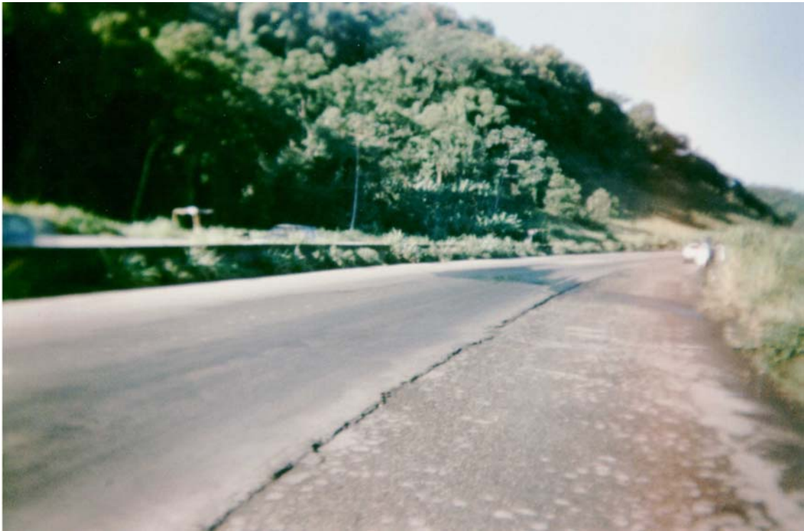
View of a BR-277/PR segment with water emerging on the revetment (January 1999)
