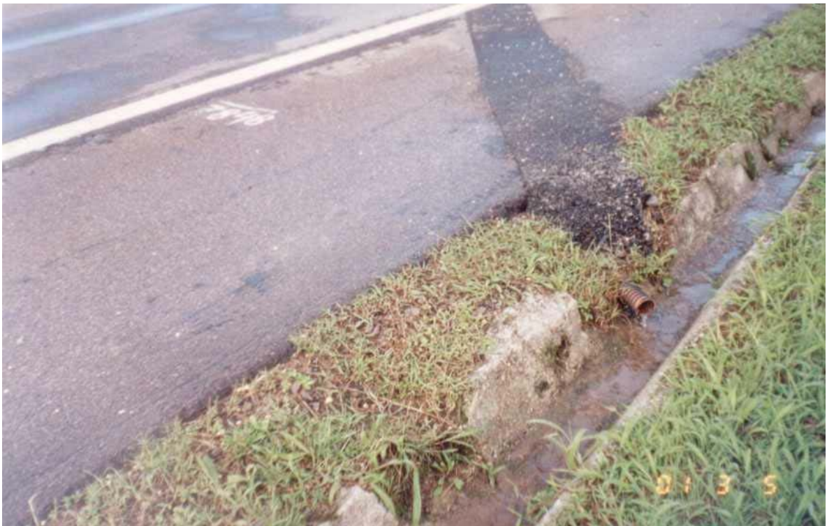
Detail of a transversal drain implemented with desembogue direct to the gutter
