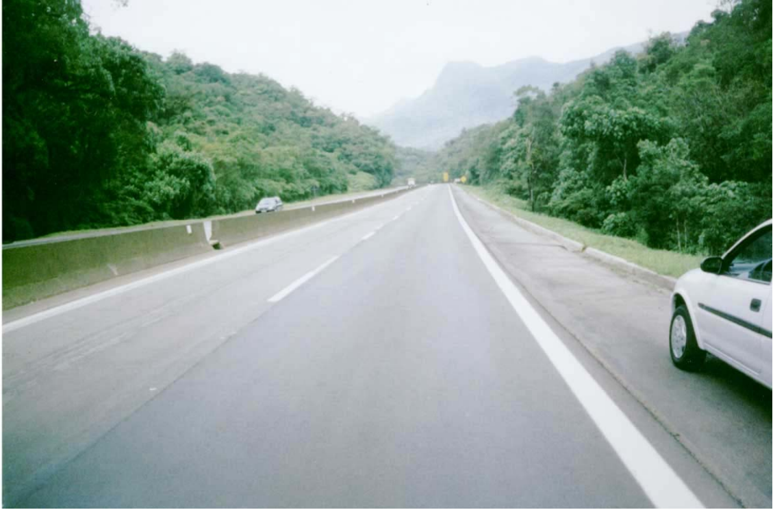
Detail from the local, placed in a segment that suffered intervention with the implementation of pavement drain and pavement restoration (November 2003)
