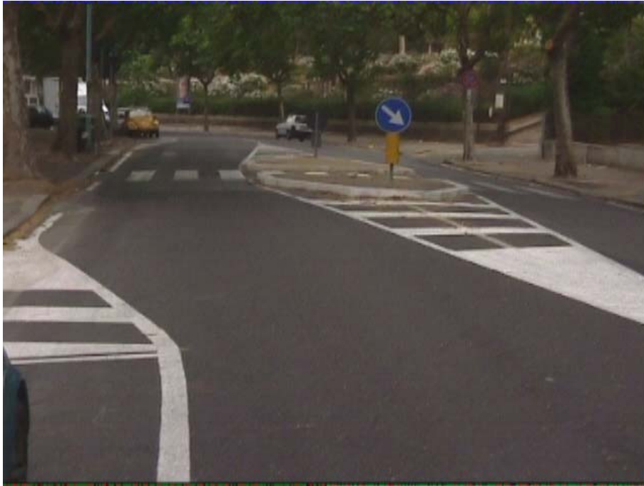
Figure 8: View of the new crossing point
