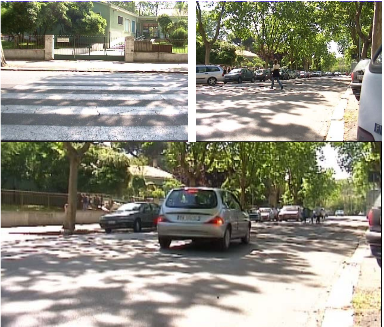
Figure 3: The crossing point (station 1) before the renewal
