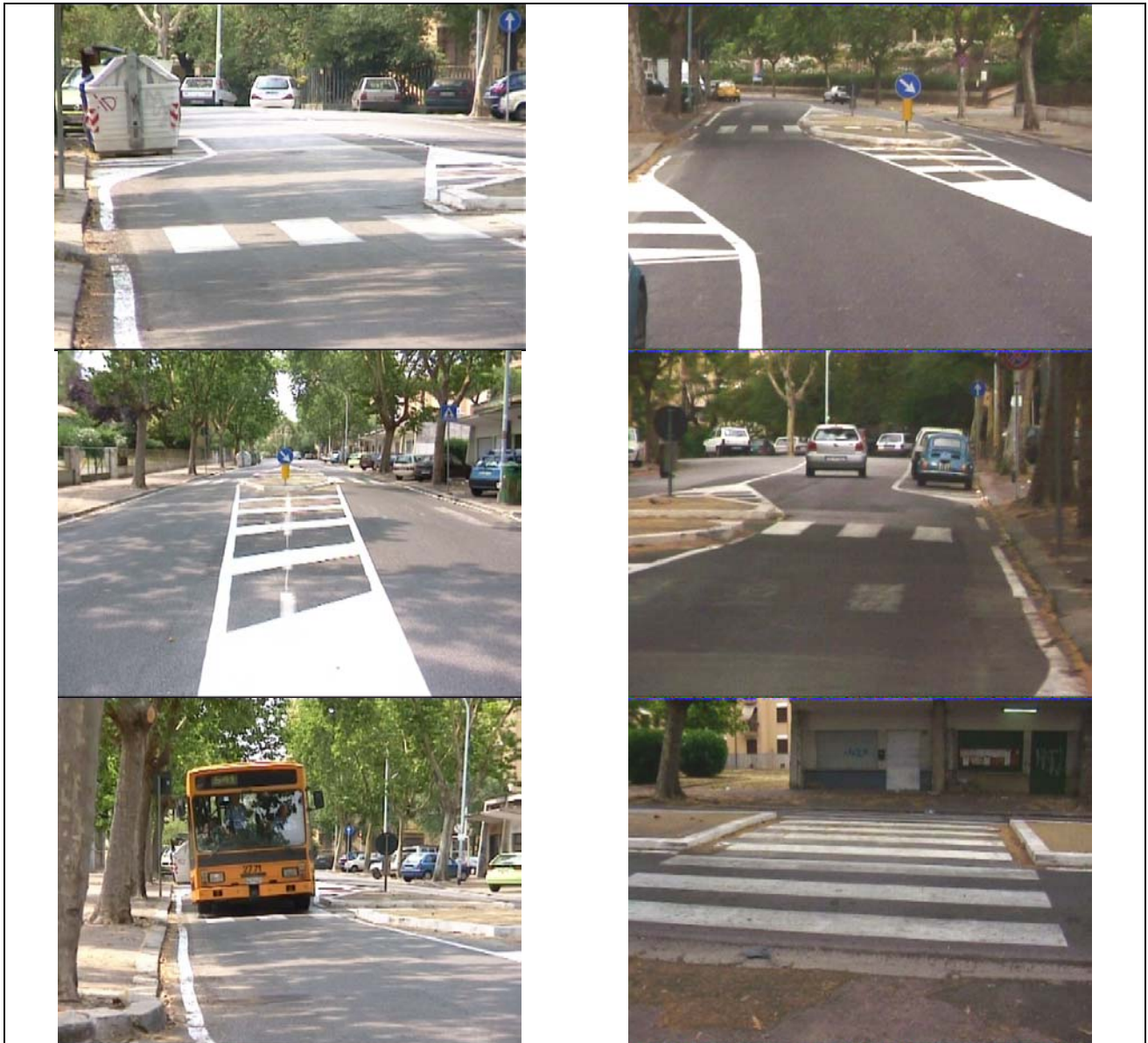
Figure 7: Views of the new crossing point
