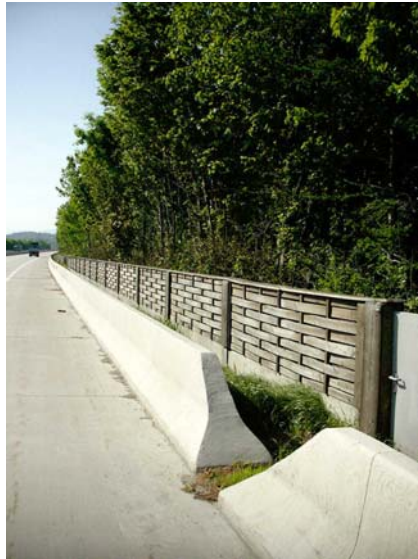
Figure 2: the formerly existing noise wall
