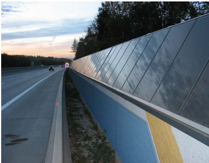
Figure 4: the new wall with integrated photovoltaics
