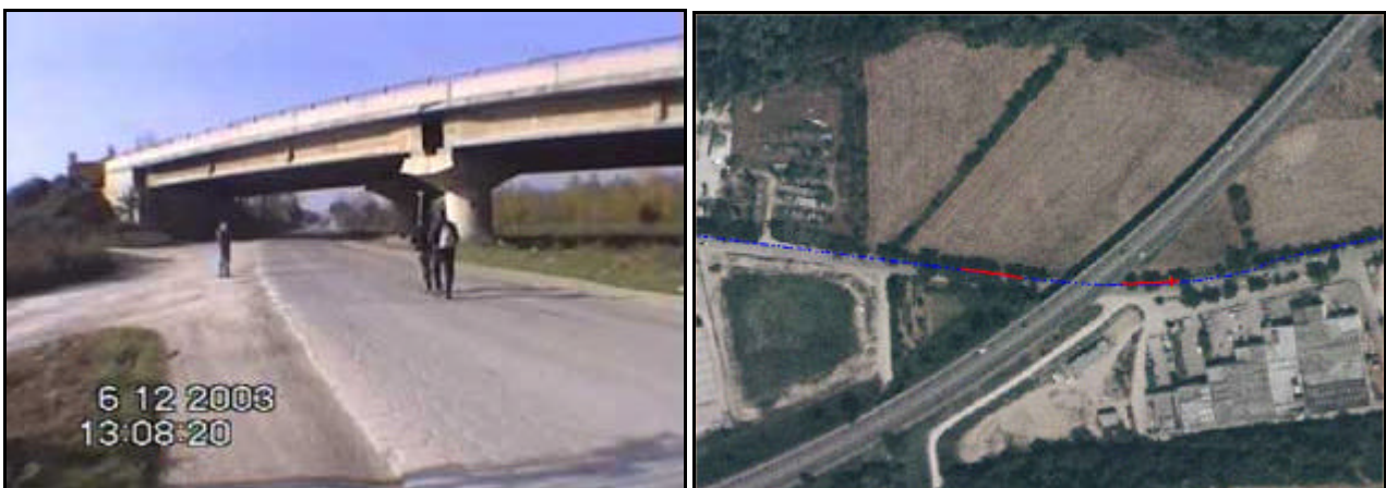
Figure 7: The road axis repeatability. Left: survey process; Right: evaluation
