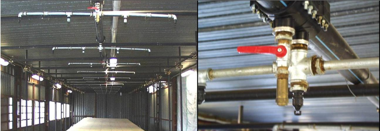
Figure 10 – Transversal lines of pipes and particular of nebulizer CENTURION and sprinkler FULLJET.
