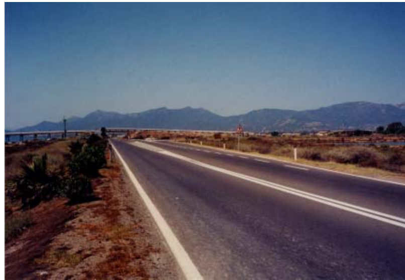
a) Identification of the intervention visual area: the intersection at the Enichem jetty.
