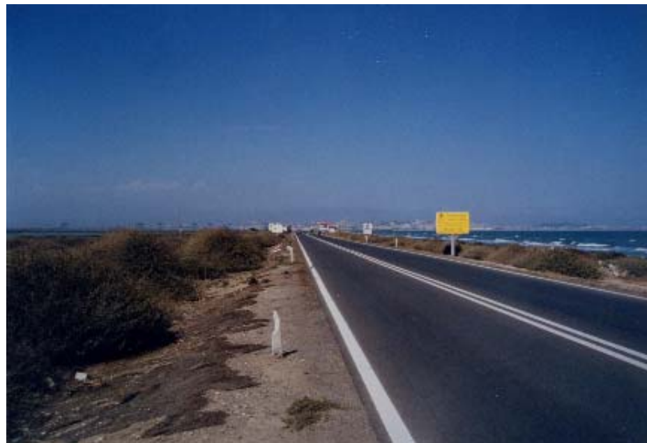
a) Identification of the intervention visual area.
