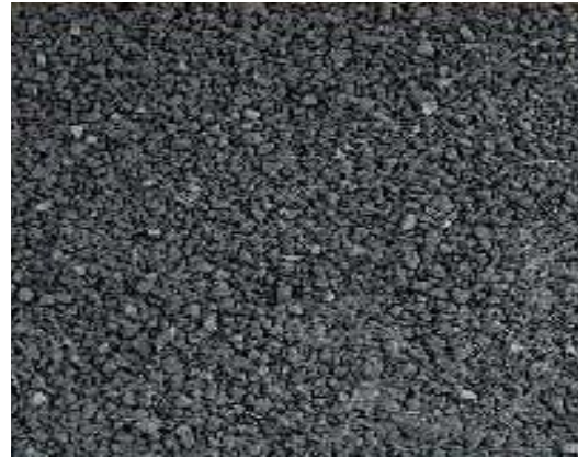
Figure 7: The lack of compactness of the second mix
