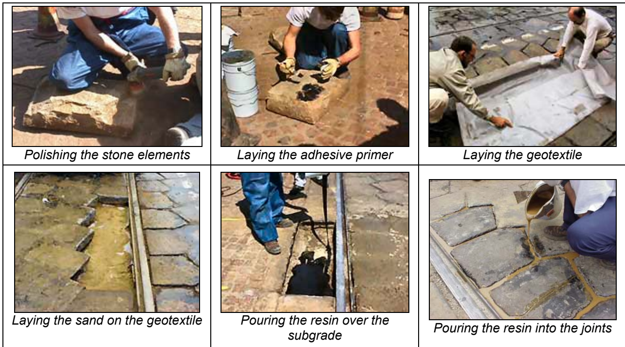
Figure 12. Installation of the stone elements with the new technique
