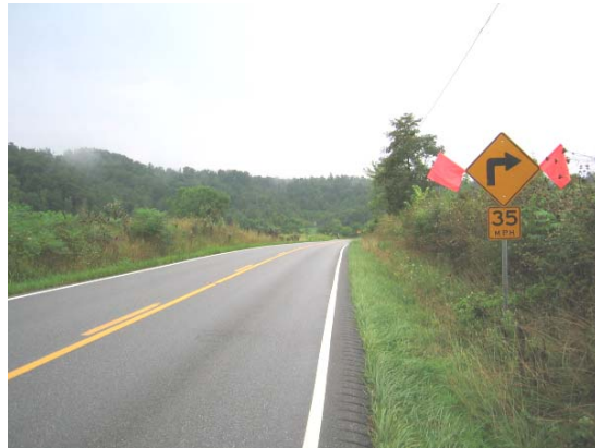
Warning sign with flags
