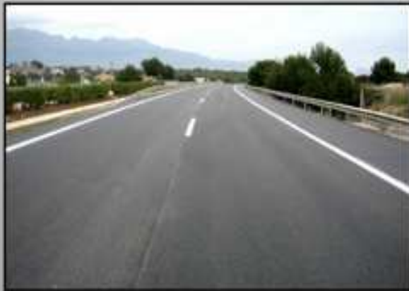
1,250 waste tyres used per lane kilometer in a 50 mm overlay
