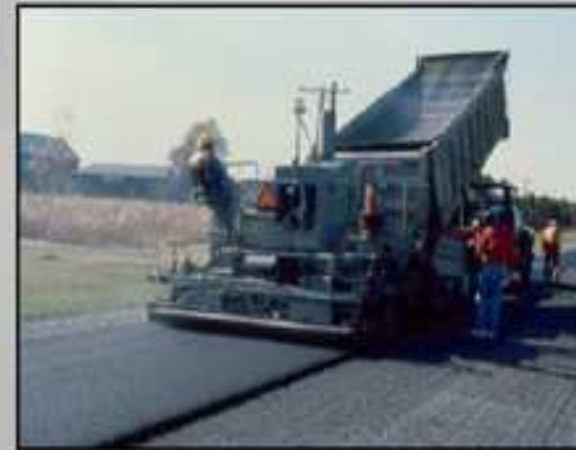
Asphalt rubber is used in a typical paving procedure
