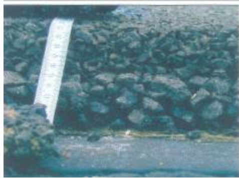
Figure 7: View of a typical composition of the double layer in a trial section laid in Italy (La Torre et al, 2002).
