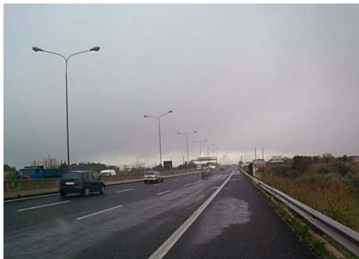
Figure 5: Typical example of the failure of a project
