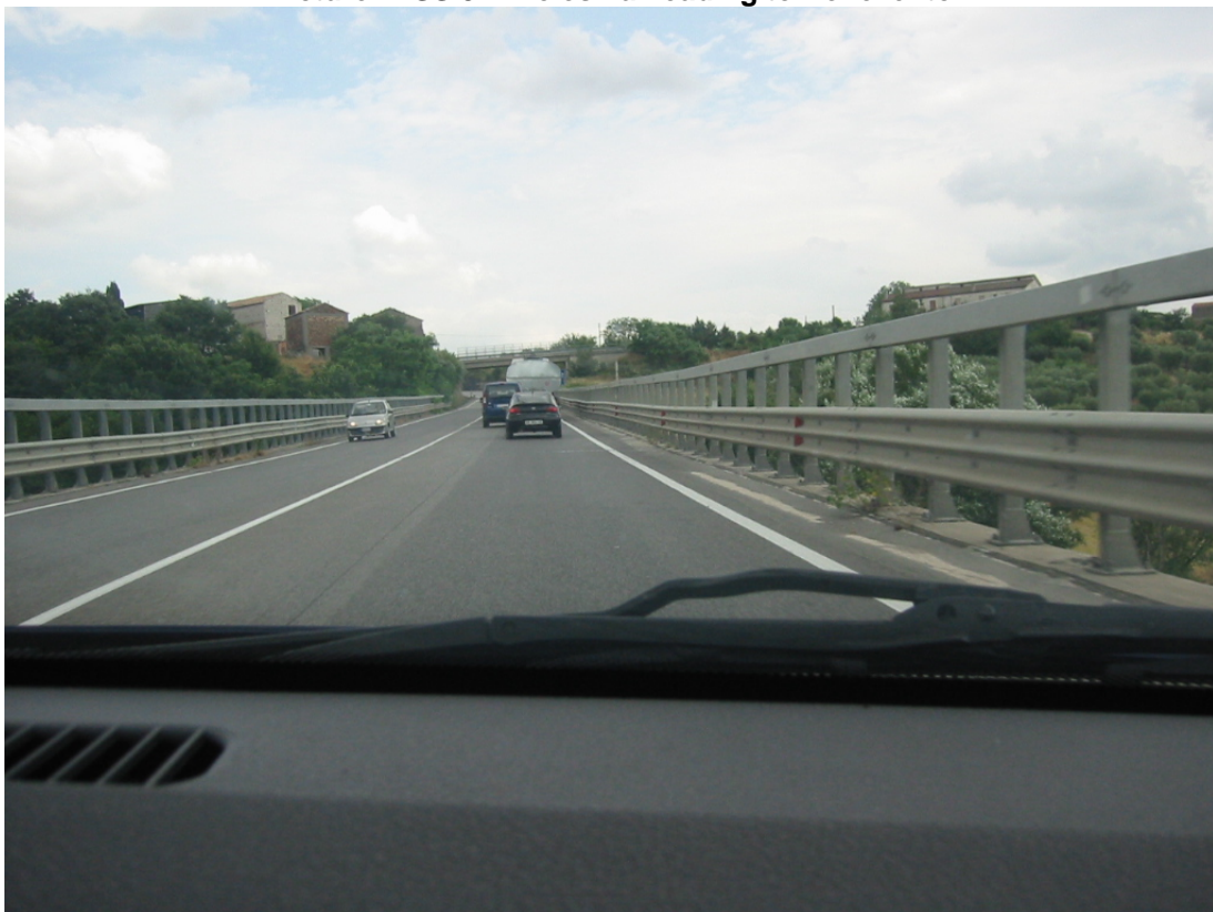
Picture 1: SS 372 Telesina heading to Benevento
