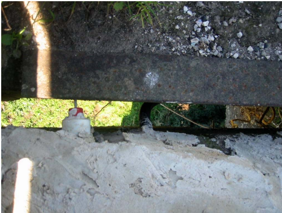
Picture 3: linear expansion joint gauge installed
