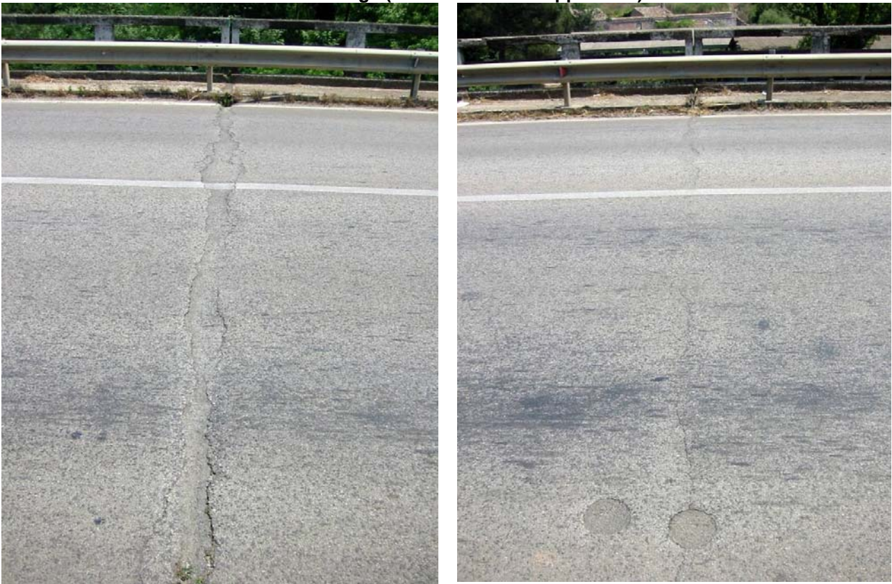
Picture 2: unusual displacement of the expansion joint on the first deck of the Savone bridge (as seen from the upper side)
