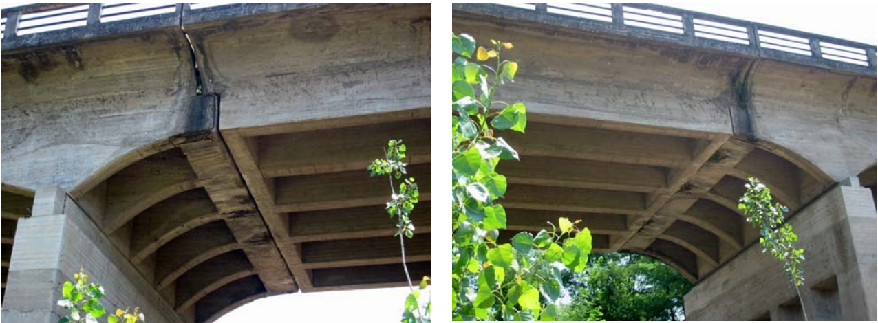
Picture 1: unusual displacement of the expansion joint on the first deck of the Savone bridge
