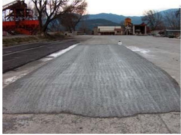
Fig. 3: Superficial finishing at the end of laying
