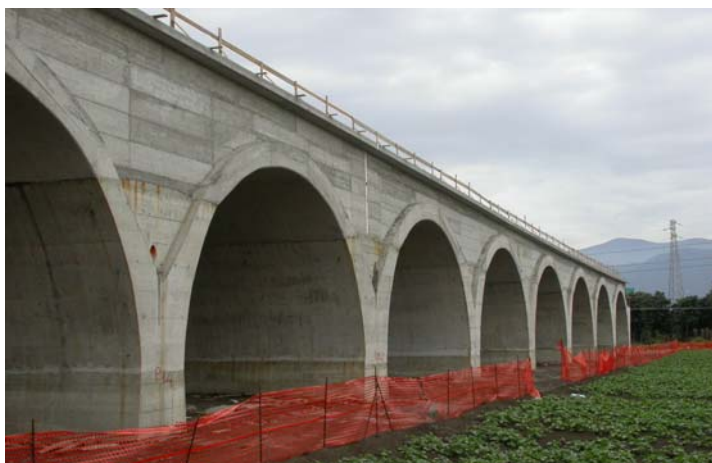
Figure 14: View of spans
