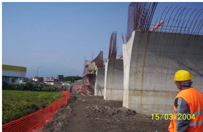
Figure 11: View of piers
