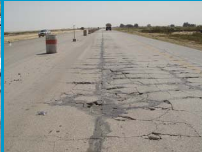
(fatigue) cracking of bound layers
